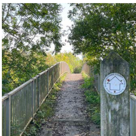
Existing A10 Bridge:
